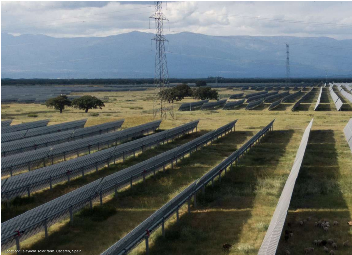
Location: Talayuela solar farm, Cáceres, Spain
